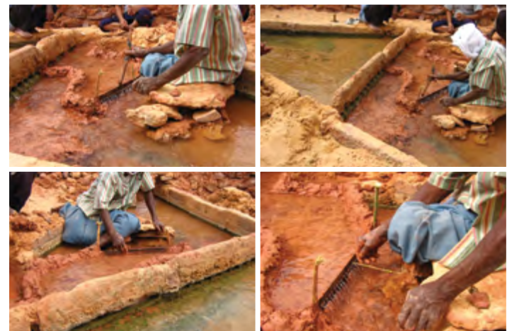
Traditional techniques for foggara maintenance in the Adrar. Photo: Taha Ansari, 2010.
