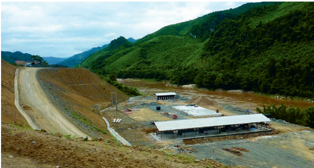
Construction Site of the Xayaburi Dam
