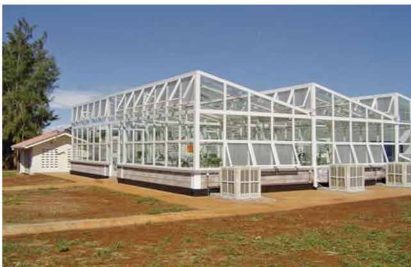
Plate 3. Biosafety level 2 greenhouse facility at Kenya Agricultural and Livestock Research Organization (KALRO), Kenya. African governments should invest resources in infrastructural development of such facilities to enhance research in modern biotechnology.
