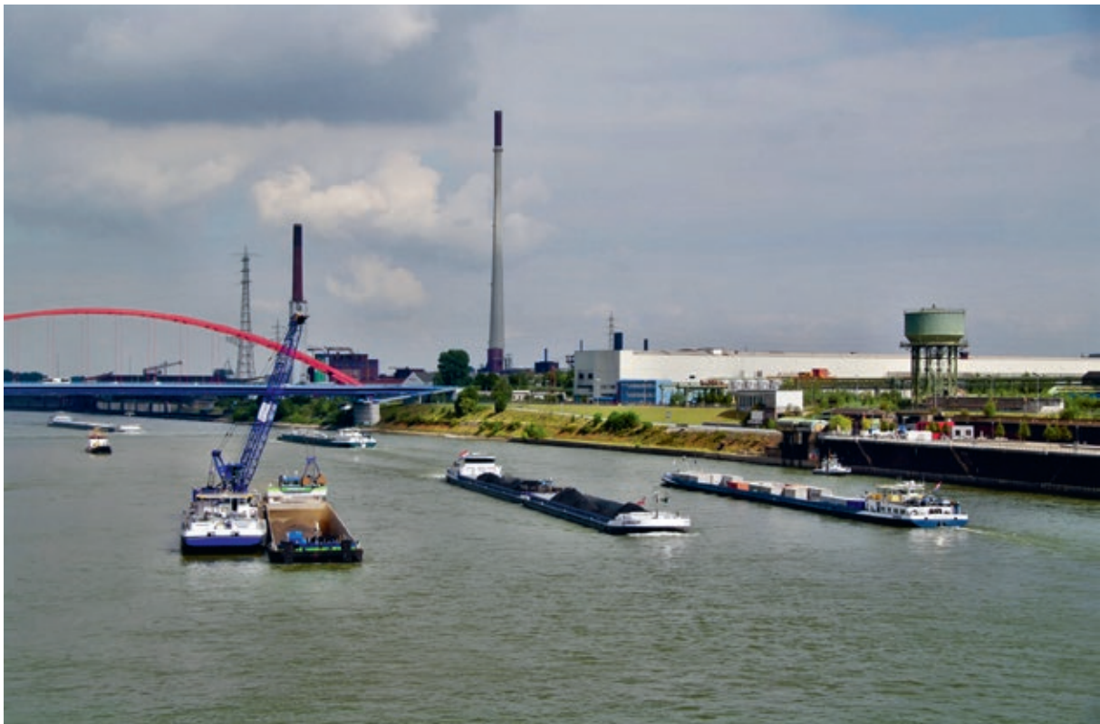
The Rhine River and its water are used for multiple non-competing demands: transportation, hydropower, cooling water for thermal power plants, industrial process water, withdrawal of bank filtrate for drinking water supply, tourism.
